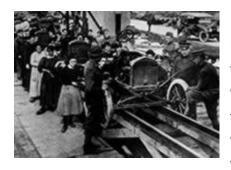
Parts were attached to a moving Model T chassis in order, from axles at the beginning to bodies at the end of the line. As vehicles moved past the workers on the line, each worker would do one task. Some components took longer to put together and attach than others. Subassemblies were established for these. For example, each
